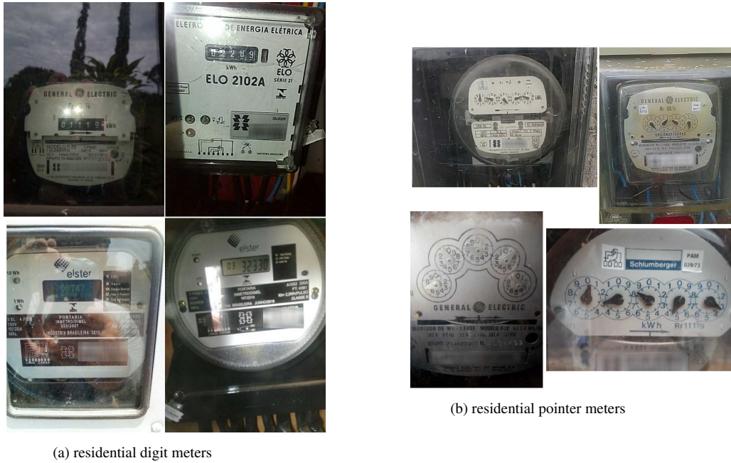
Figure 1.1: Examples of residential meters.
